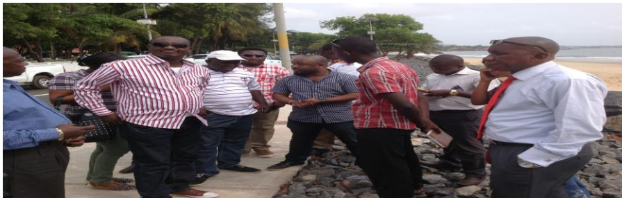
Committee Members inspecting Lumley-Aberdeen road project.
